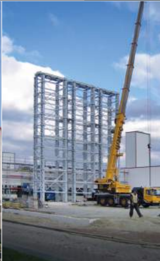
Capacity: 61 cassettes / L 3,500 mm, T 800 mm, H 240 / 480 / 640 mm Payload per cassette: up to 5,000 kg Machine dimensions: H 20,500 mm, W 4,500 mm, D 3,400 mm
